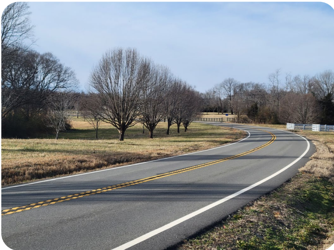
Below: Existing road and pedestrian networks in Cumberland County.
