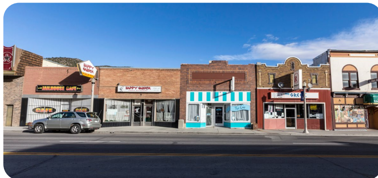
Small town brick storefronts along historic Ely, Nevada, USA.
